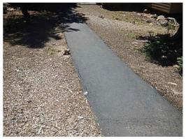
300 - Asphalt: Overlay w/ Interlayer Useful Life 25 Remaining Life 6
